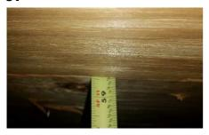
Location: Throughout System: Wind Mitigation Condition: Photo Of Plywood Thickness Explanation: Field Measurment Impact Consequences: NA Recommended Action: NA
