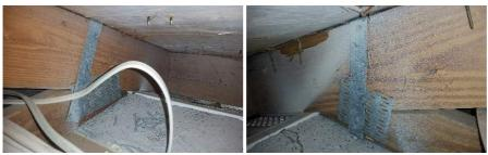
Location: Throughout System: Wind Mitigation Condition: Photo showing detail of a Single Wrap Detail Explanation: Single Wraps Metal Straps must be secured to every rafter and or truss with a minimum of 3 nails wrapping over and securing to the opposite side of the rafter and or truss with a minimum of 1 nail. The Strap must be attached to the top plate of the wall frame or embedded in the bond beam in at least one place. Impact Consequences: No Comment Recommended Action: No Comment
