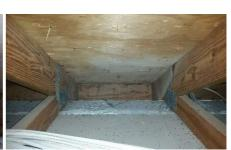
Location: Throughout System: Wind Mitigation Condition: Photo showing detail of a Single Wrap Detail Explanation: Single Wraps Metal Straps must be secured to every rafter and or truss with a minimum of 3 nails wrapping over and securing to the opposite side of the rafter and or truss with a minimum of 1 nail. The Strap must be attached to the top plate of the wall frame or embedded in the bond beam in at least one place.
